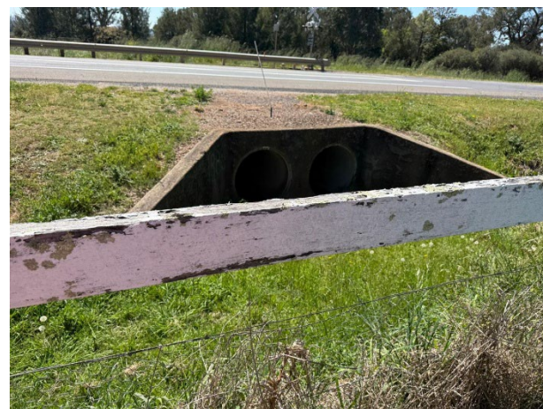
Image 4: Dual concrete culverts along the southern boundary of Lot 2, aligned parallel to the railway track. No water flow was observed during inspection.
