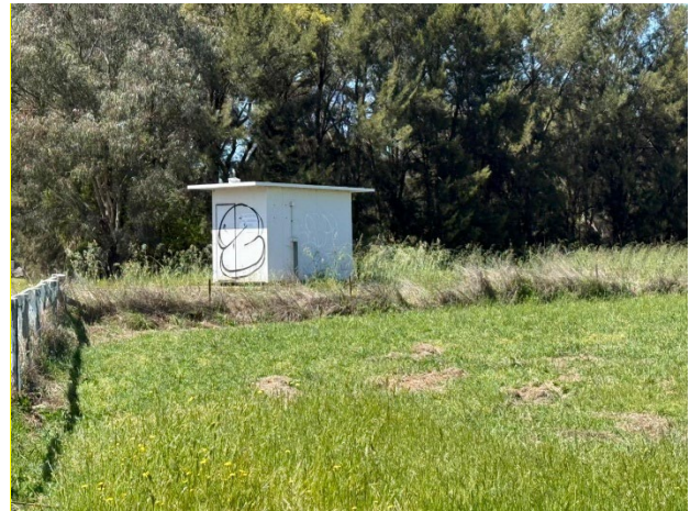
Image 6: Utility shed near railway line may be associated with storage or service (not in the property).
